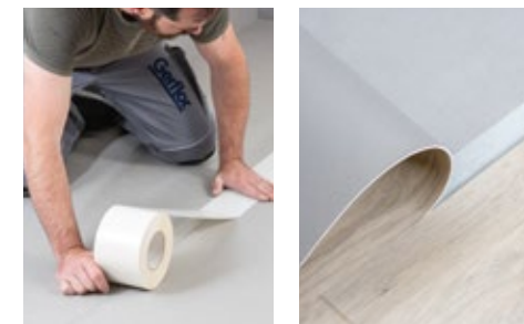
2. Place the hop holding tape and position rolls
