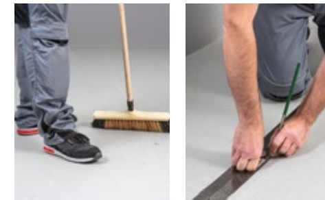
1. Clean the subfloor and mark the position
