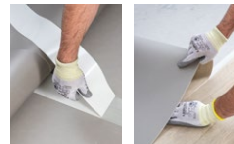
3. Remove the protective film and unroll the flooring
